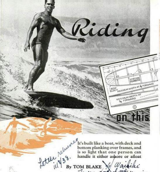
YOU'LL get plenty of thrills when you try this speedy hollow surfboard, either riding the waves of the open ocean, freeboard aquaplaning in the wake of a speedboat, sailing or just paddling about on fresh-water lakes. It's nothing more or less than a shallow pontoon, light, structurally strong and virtually unsinkable. So great is the safety factor that it has been officially adopted in many localities as standard lifesaving equipment.
