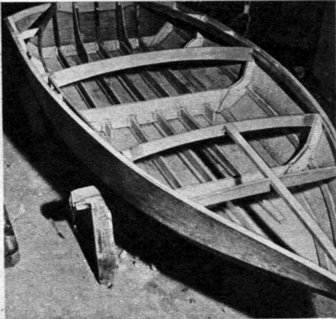
Deck framing completed, it's now ready to receive 1/8" plywood decking. Stringers go through frame 2.
