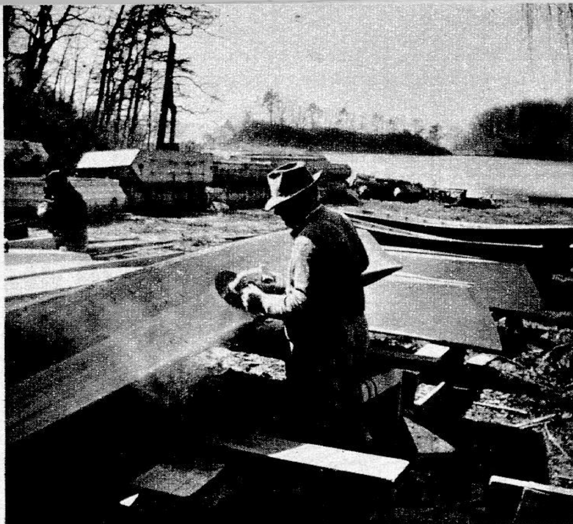
To impart in jigtime that mirror-smooth finish that we all admire on a fine boat, use a power sanding machine.
